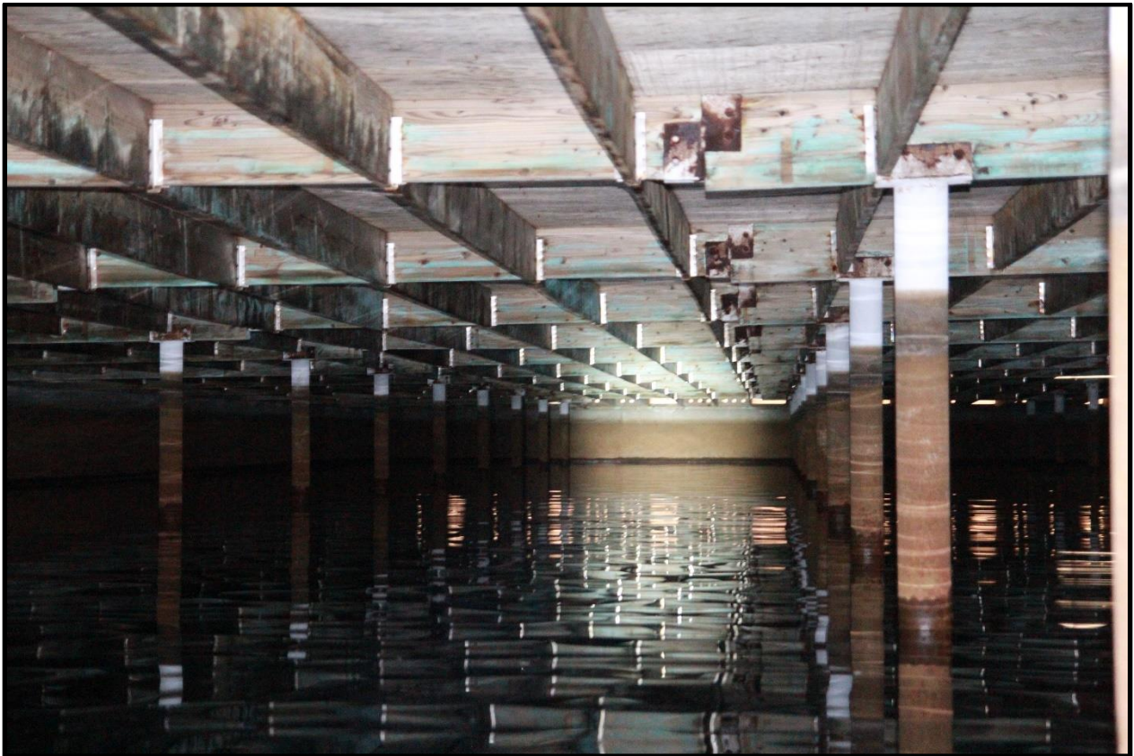
Reservoir Roof Structure
