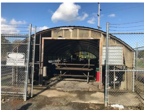
7 Storage Area / Shed
