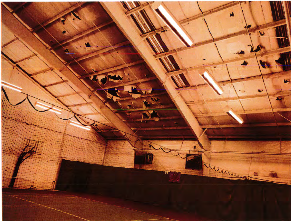
Ceiling conditions over courts 1 and 2.
