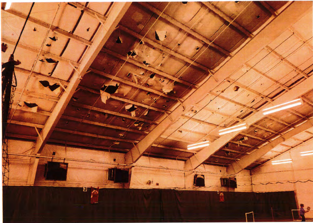
Ceiling conditions over courts 3 and 4.
