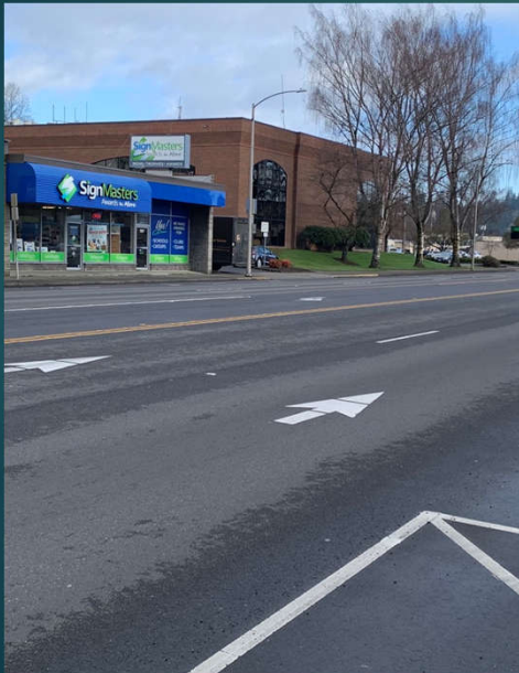
15 th Ave Resurfacing
