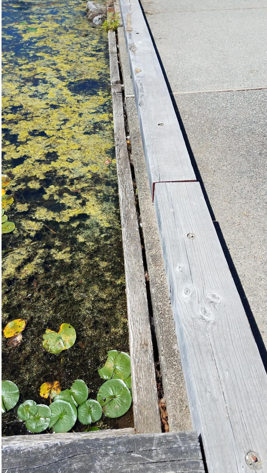
Martin's Dock - face board and wood rail
