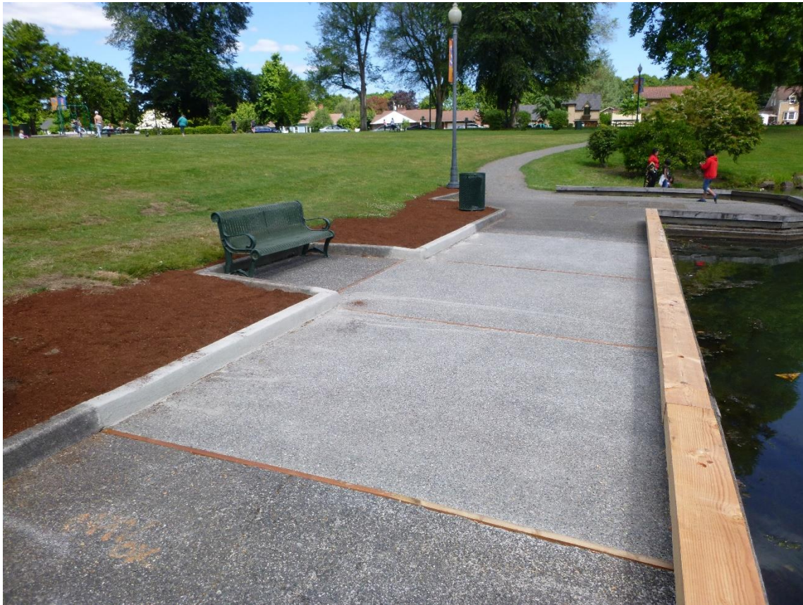
Martin's Dock – panels, wood rail and expansion joints replaced in 2018
