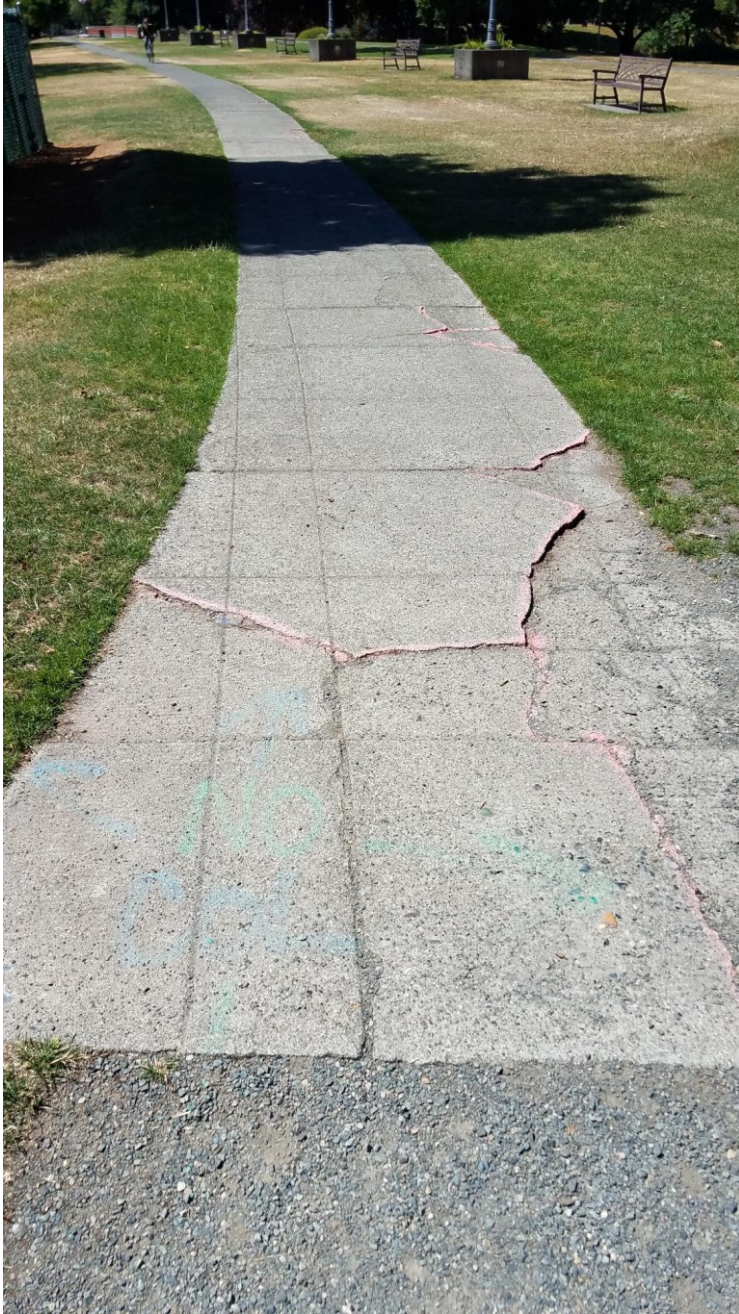
Photo # 1: South side of the sidewalk start of project
