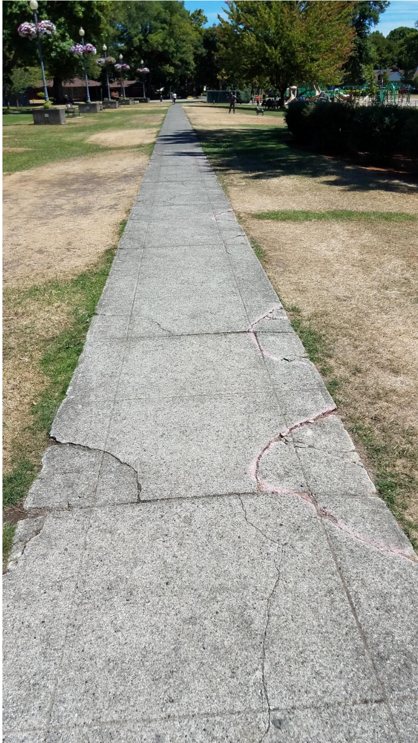
Photo # 2: South side of the sidewalk
