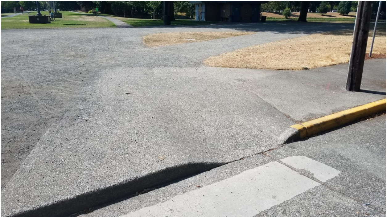
Photo # 15: NW ADA ramp
