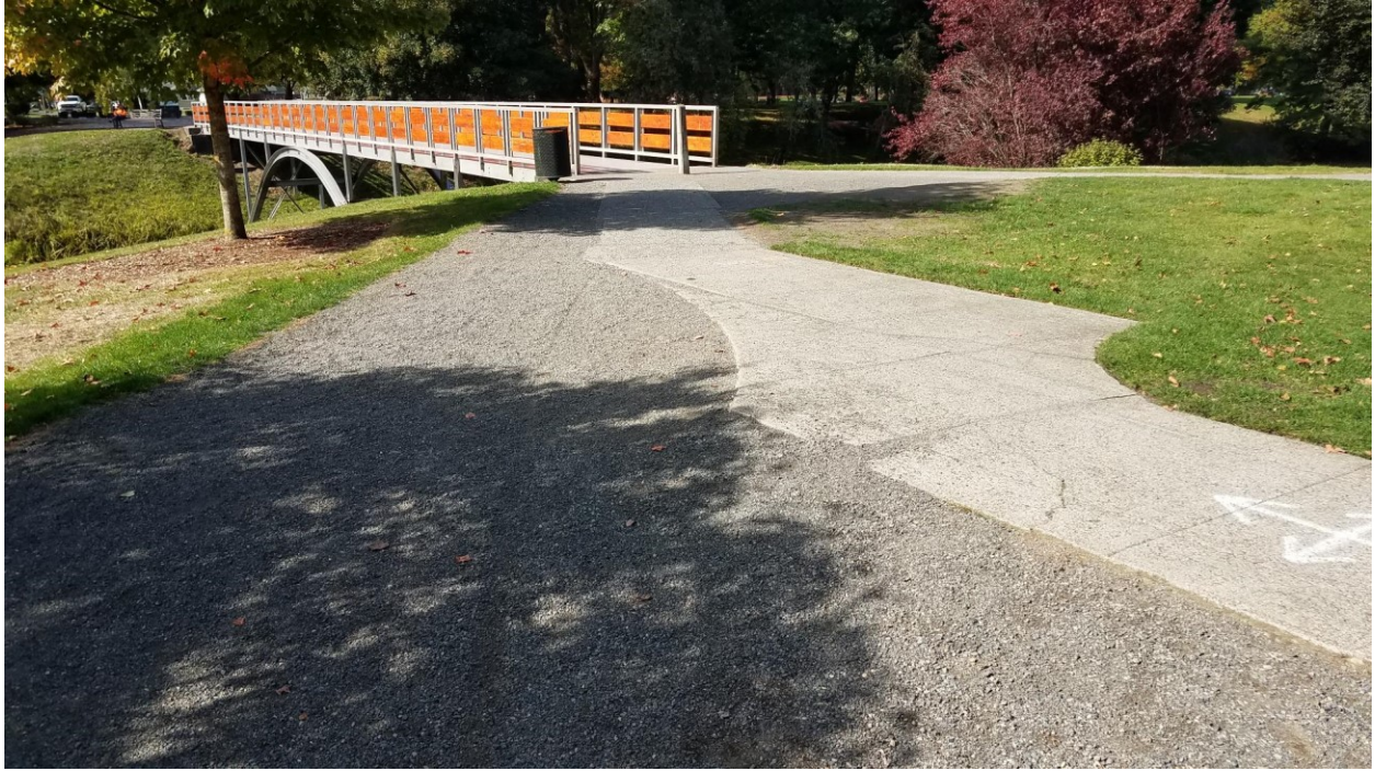
Photo # 3: South side of the sidewalk near the pedestrian bridge and path leading south
