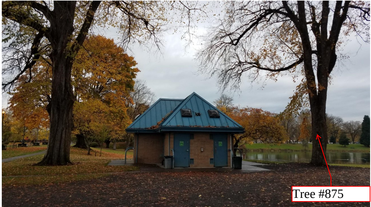
Restroom – east side overview
