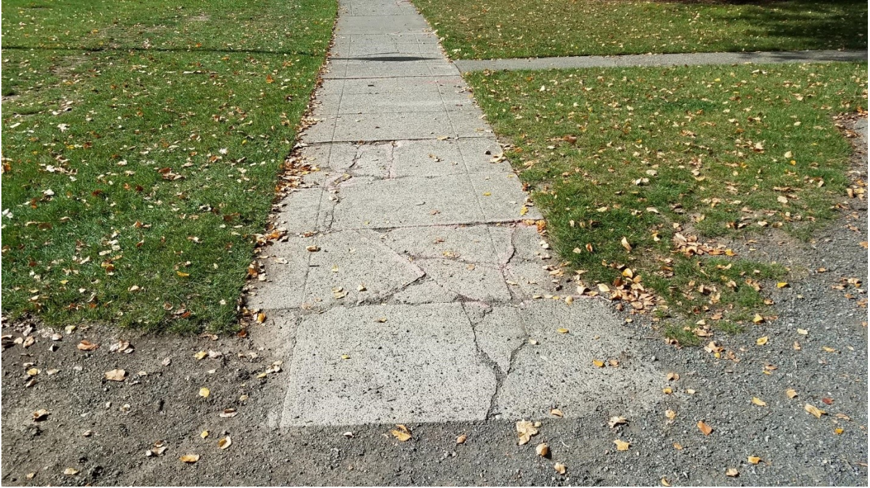
Photo # 7: North side of the sidewalk end of project
