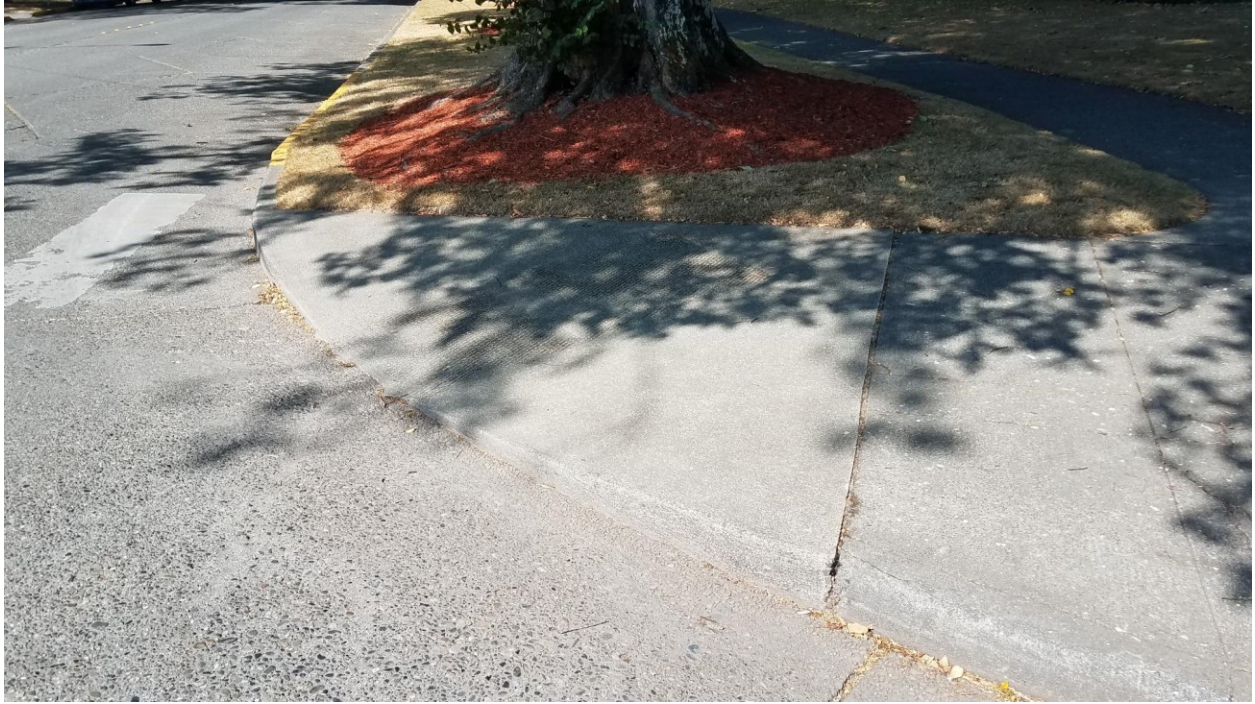
Photo # 14: NE ADA ramp
