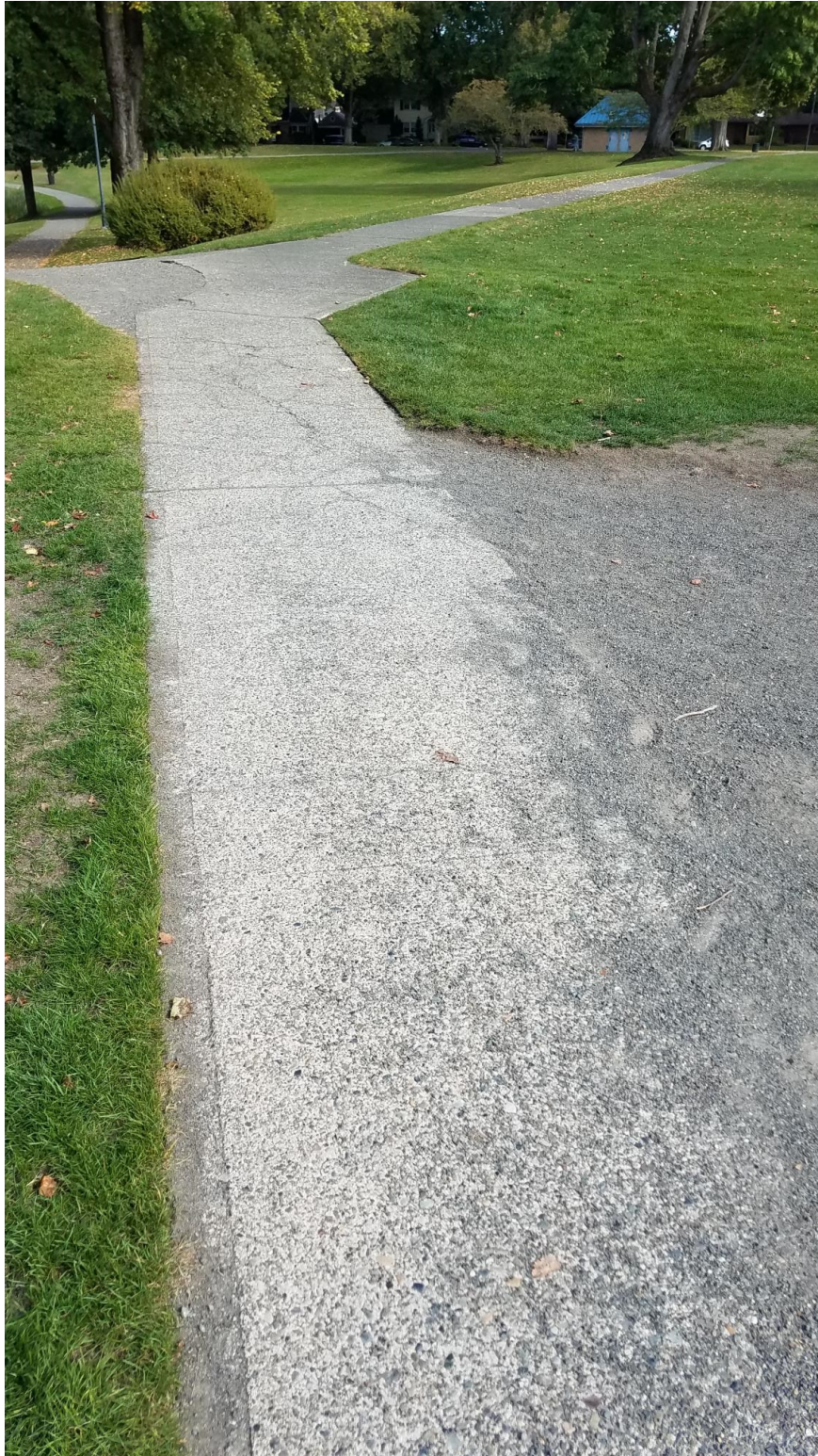
Photo # 5: North side of the sidewalk near the pedestrian bridge leading to the trail north
