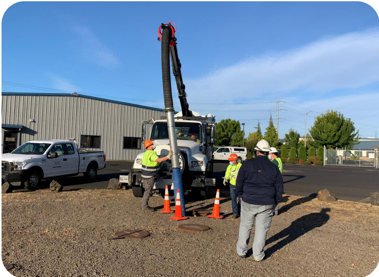
Maintaining a City-owned Stormwater Treatment Vault in 2021
