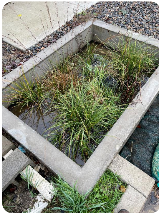
Filterra Bioscape Vault Installed at a New Residential Subdivision in 2021
