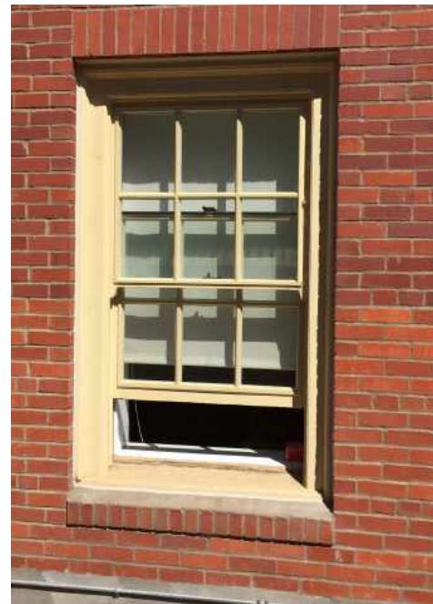
Window with SLIP attachment added
