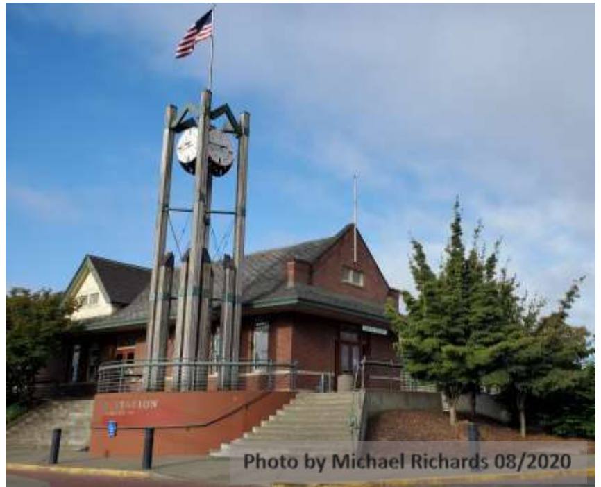
Figure 5 Kelso Train Depot
