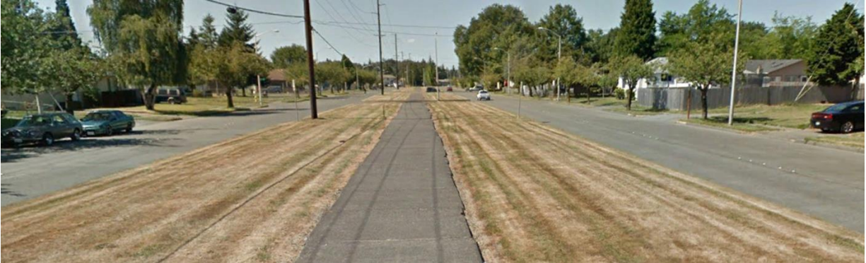
Beech Street today 2 two-lane, one-way streets With a box culvert in the middle.
