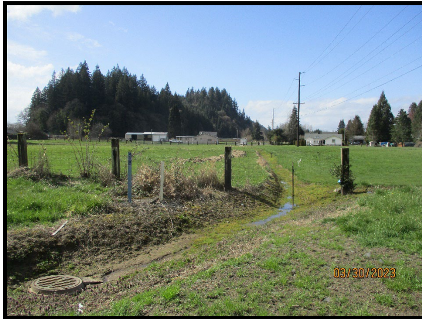
Photograph 3: Non-jurisdictional drainage ditch running along the northern boundary of the subject site. Water from this ditch flows into the storm drain (lower left of photo) near the terminus of Olive Way, and thence to the Type U Diking District Drainage Ditch, which is less than 100 feet north. (Photo looking northwest from the terminus of Olive way along the western property boundary. Subject site to the left.)
