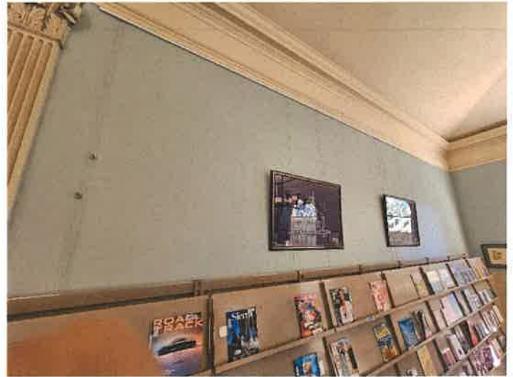
Magazine Room Existing Track Hangings
