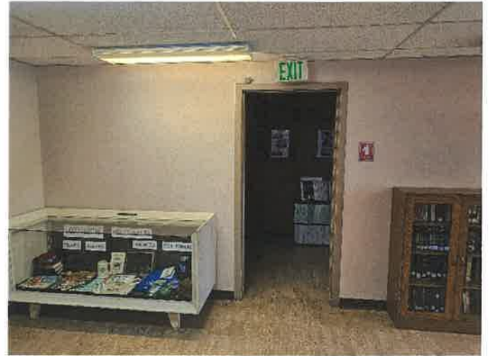
Mezzanine South Wall – Close up (1)
