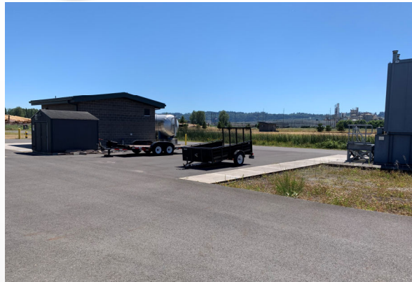
Equipment storage building $200,000
