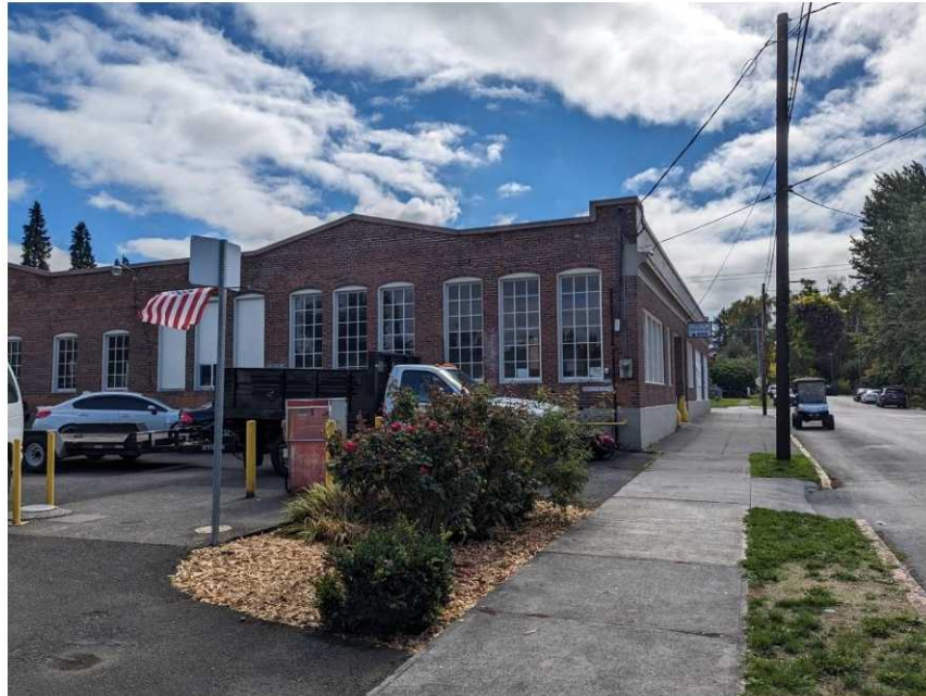
FIG 2. RSD maintenance Building, Rear
