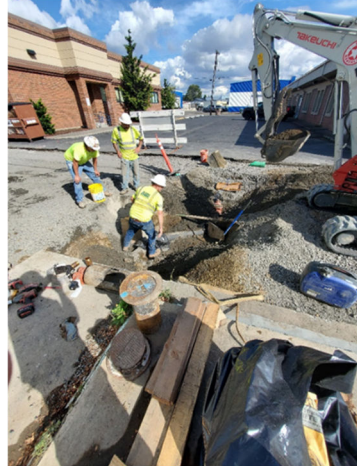
Replacement of water and sewer lines in the alley behind the Pancake House.
