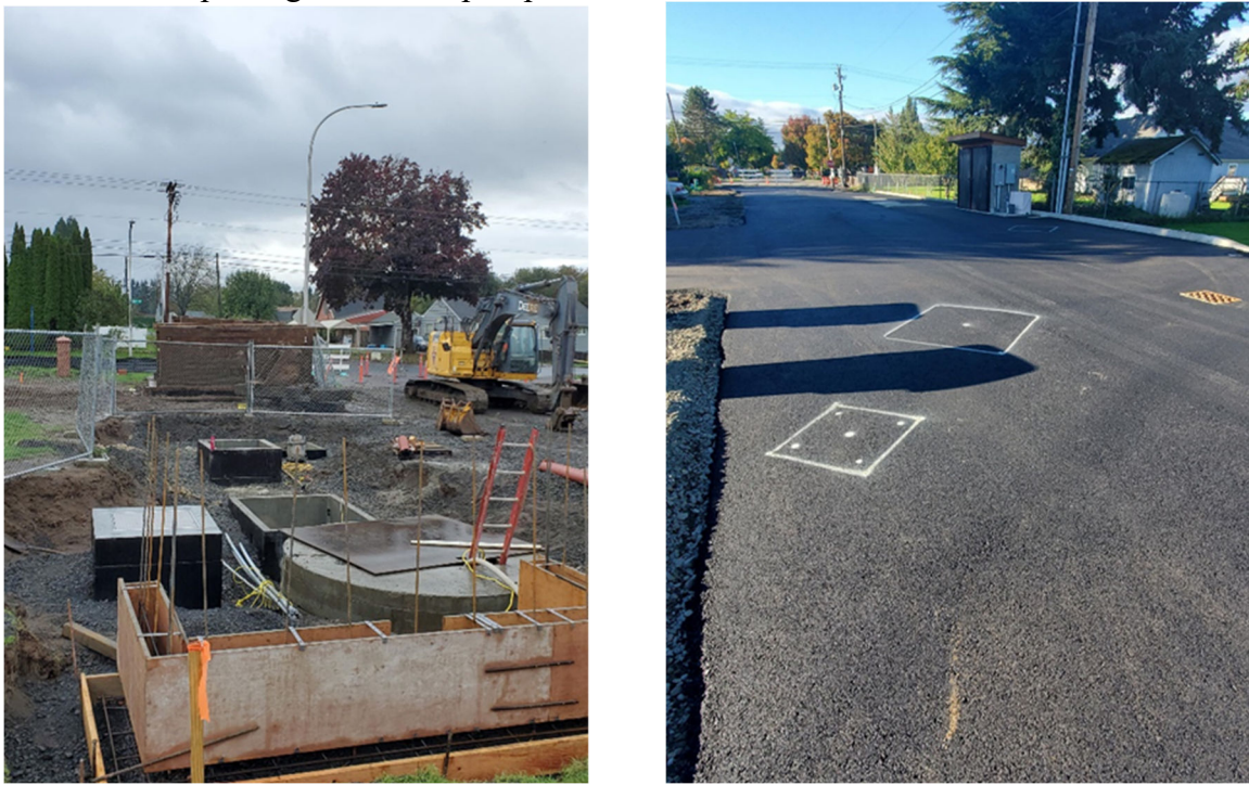
Replacing two sewer pump stations at 38 th & Penn. and 38 th & Oak
