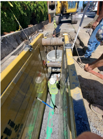
Replacement of water and sewer lines in the alley behind the Pancake House.
