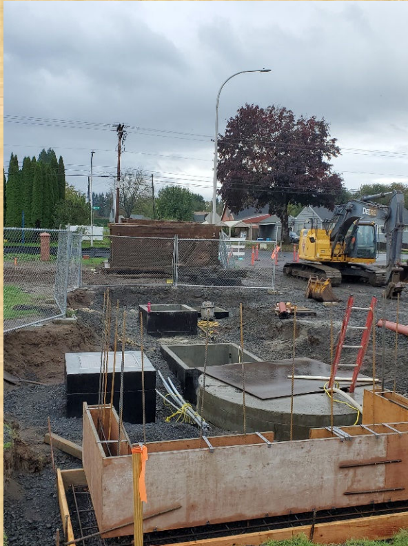
Sewer PS @ 38 th & Pennsylvania
