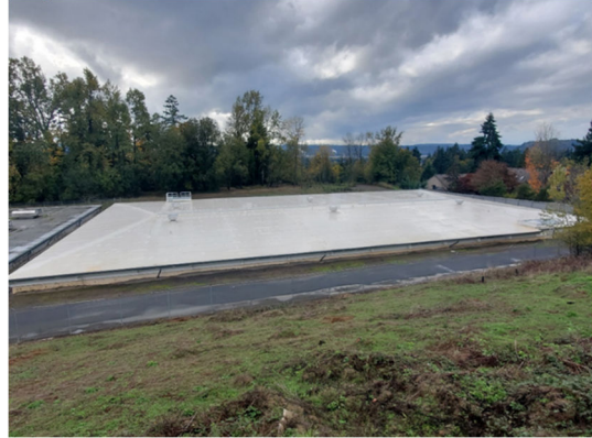
Reservoir #5 Roof Replacement
