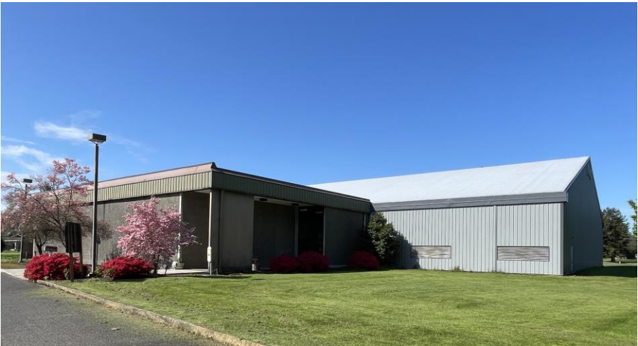
MVRC Building Exterior
