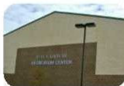
Reecy Davis Rec Center Greenville, TX
