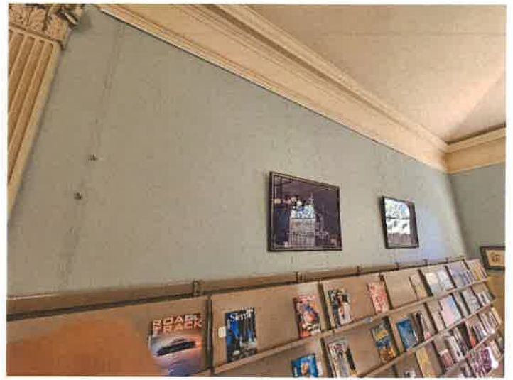
Magazine Room Existing Track Hangings
