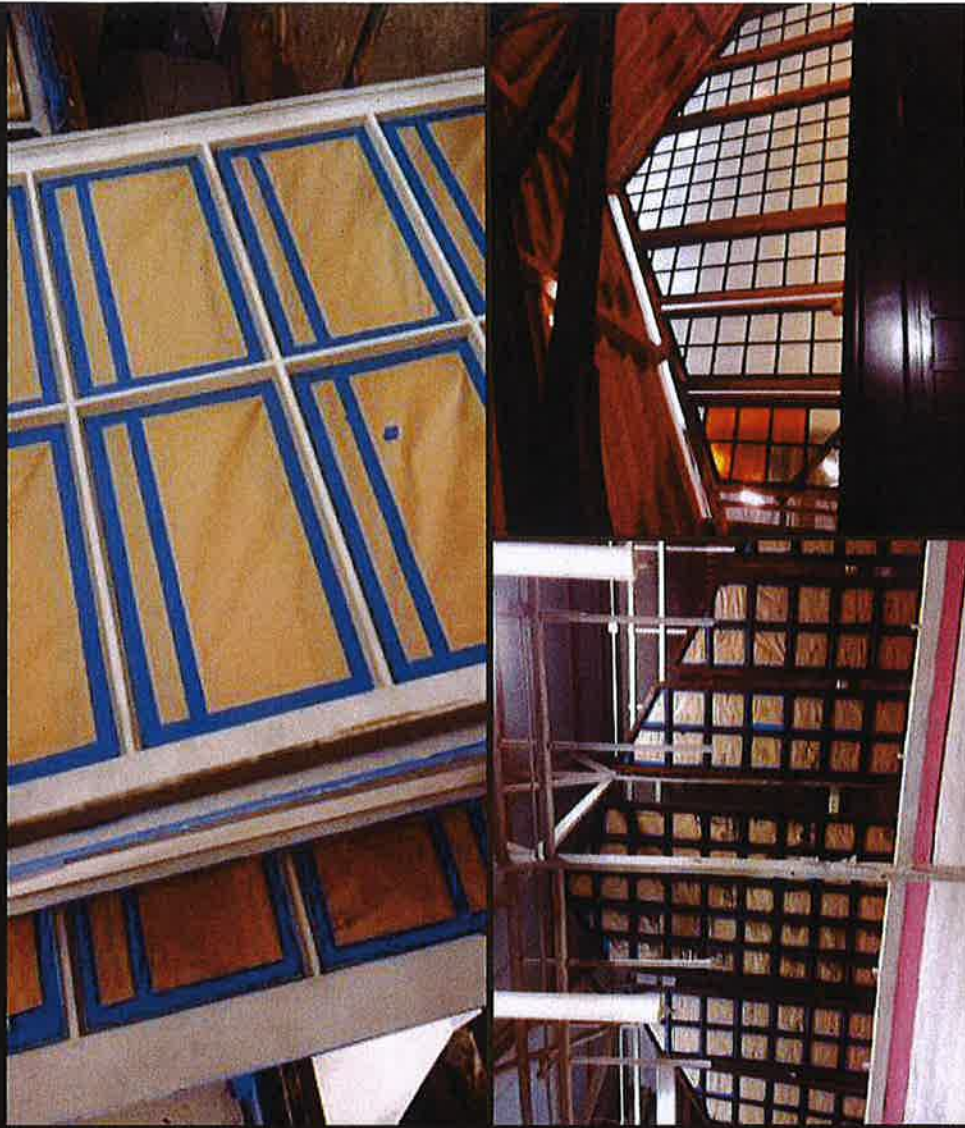
MASKING OF SASH FOR FINISH PAINT
