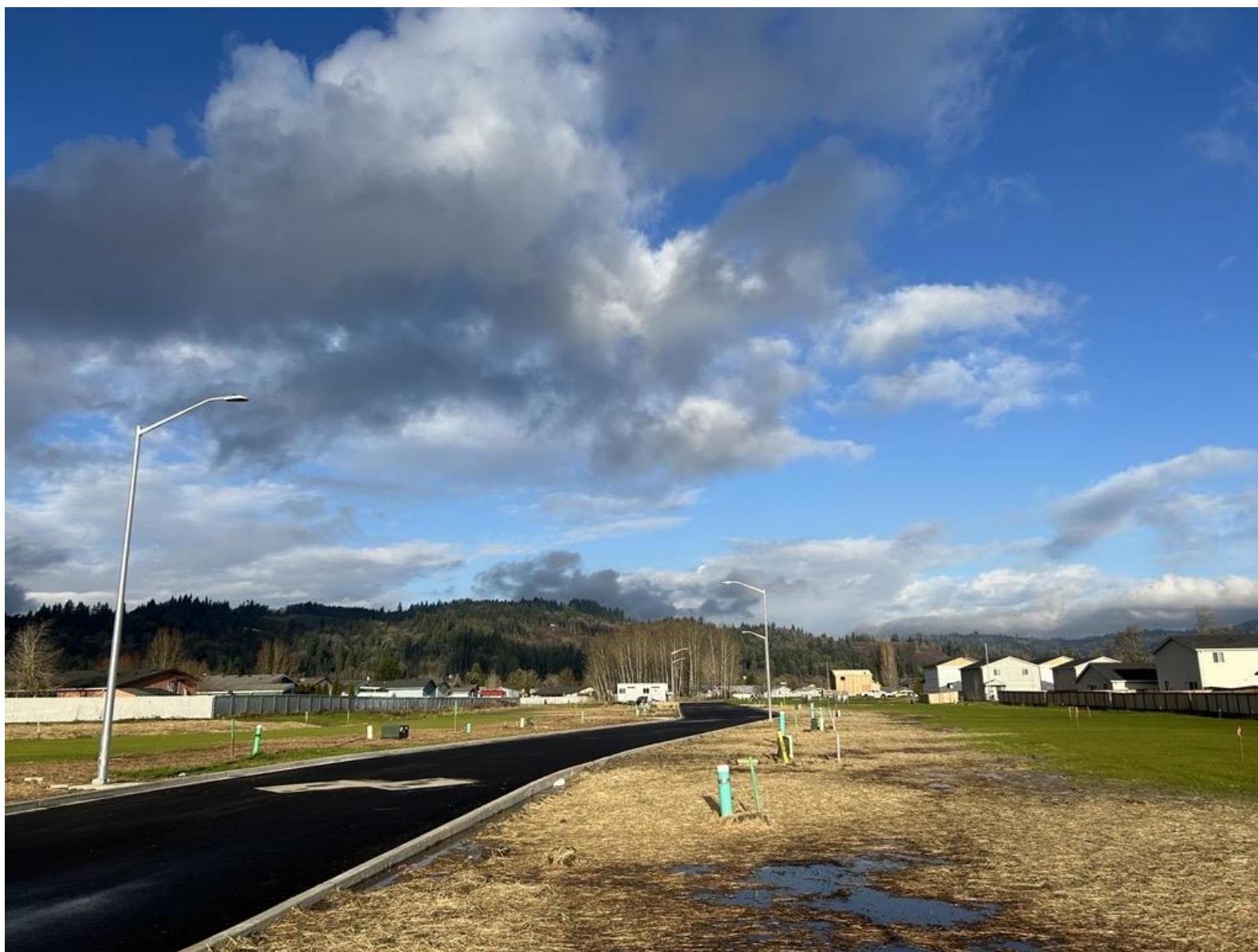
Figure 4: Looking North along Henderson Way at North end of Project
