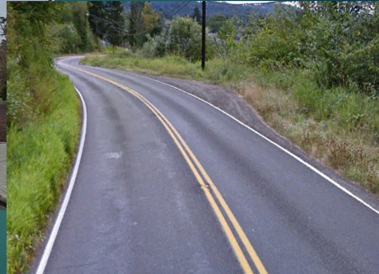
Columbia Heights 2026/2027 Construction
