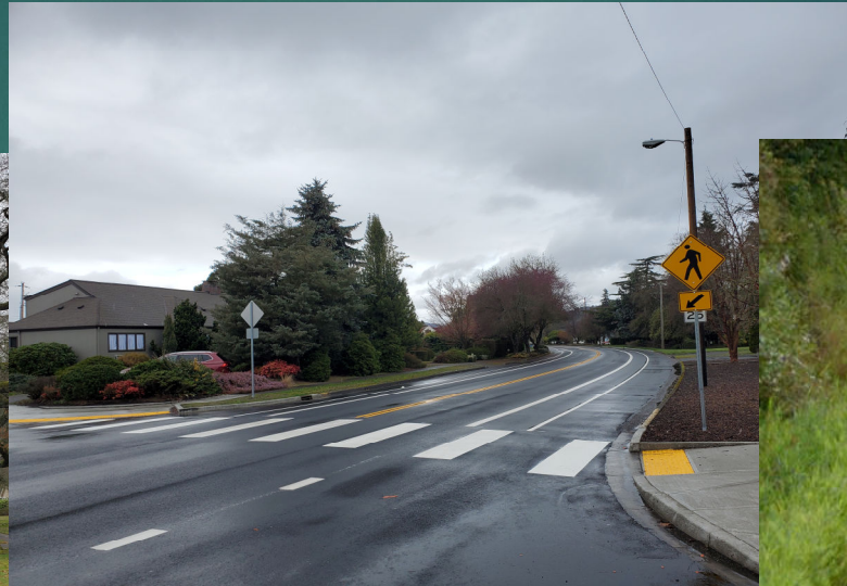
NE and NW Nichols 2024/2025 Construction
