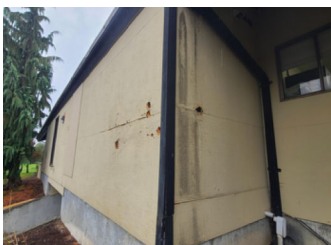
Pro Shop Siding
