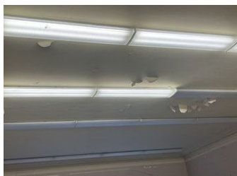
Interior restoration items
