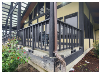
Front Porch Roof
