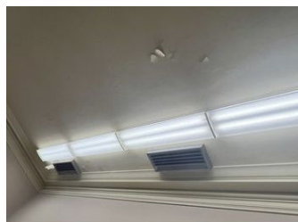
Interior restoration items
