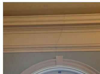
Interior restoration items
