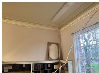
Interior restoration items
