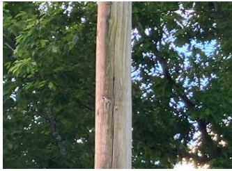
Roy Morse Light Poles - Holes
