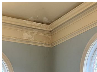
Interior restoration items
