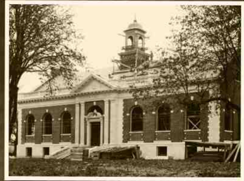
▲ Worker near the cupola during 1925 construction.
