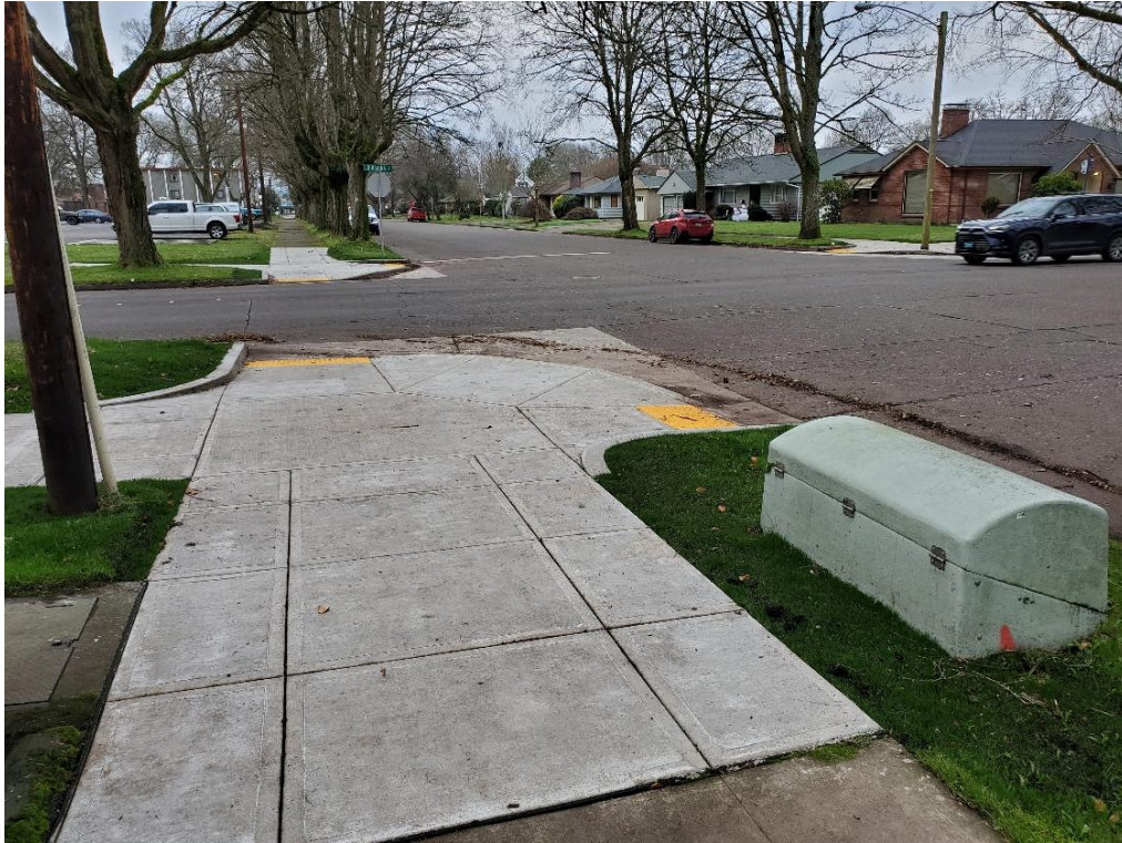
Figure 2 - 18th Ave Pedestrian and ADA crossing
